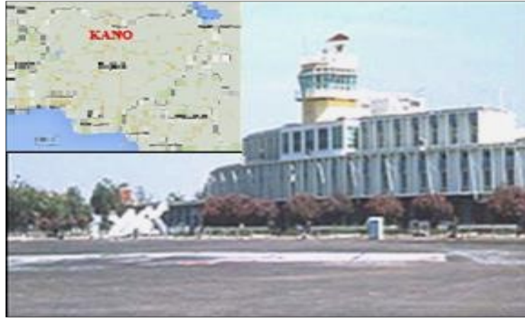
Figure 1. Location and approach view of Aminu Kano International Airport, Kano, Nigeria.
